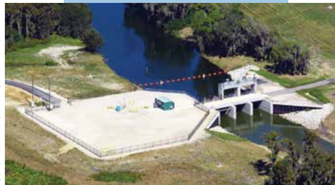
View on November 2013 of recently completed water control structure P-11 at the outlet from Lake Hancock to South Saddle Creek in Polk County.
