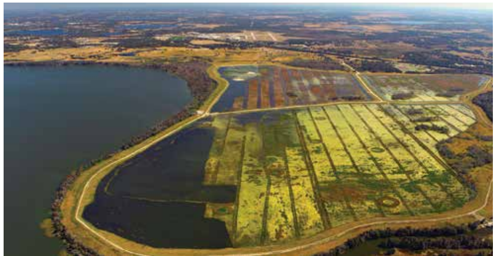
View looking east of the constructed treatment wetland located at the south shore of Lake Hancock in Polk County in January 2014.
